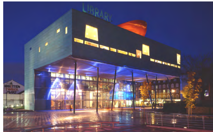
Peckham Library by Will Alsop | Source: ArchDaily.com
