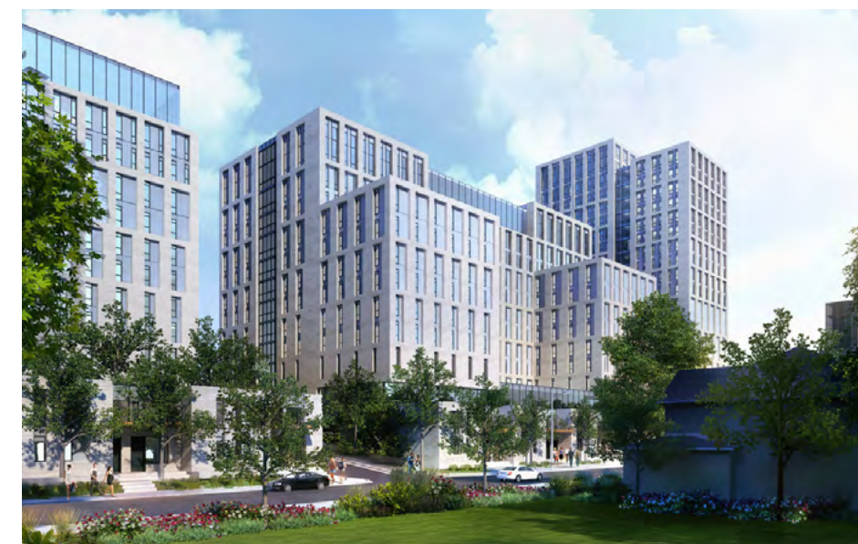
Lincoln Alexander Hall residence by Diamond Schmitt | Source: McMaster University
